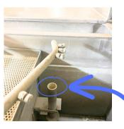
LIFT HANDLE OF DISHWASHER TO CHECK THE WATER LEVEL. THE WATER NEEDS TO BE LEVEL WITH LIP OF THIS TUBE. IF NOT, CLOSE THE COVER TO ADD MORE WATER FOR 10 SECONDS.
